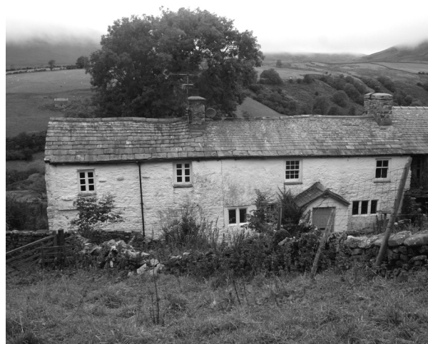
Brig Cottage, Fell End, Ravenstonedale; awaiting improvement
