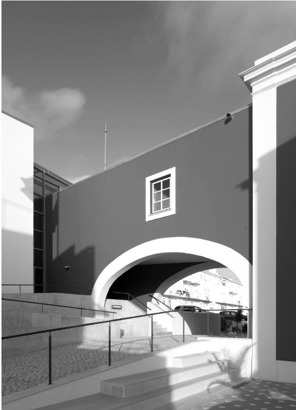
Assisted Residence, Sines
